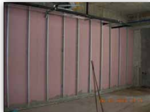
No Chasing required unlike masonry wall
