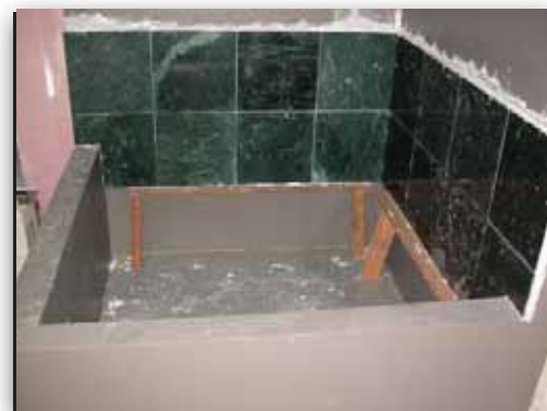
Shower area tiles/marble installed with tile adhesive.
