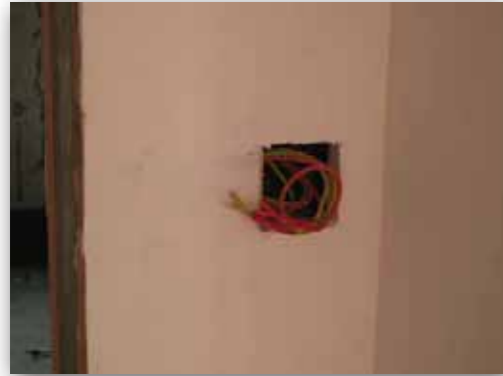
No Chasing required unlike masonry wall
