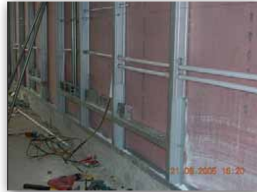
Electrical conduits easily installed in a dry wall.
