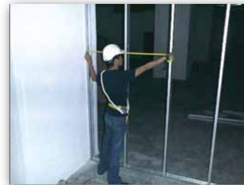
Fast erection of steel framing.
