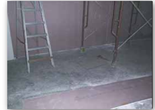
100% dry construction to achieve clean working environment.
